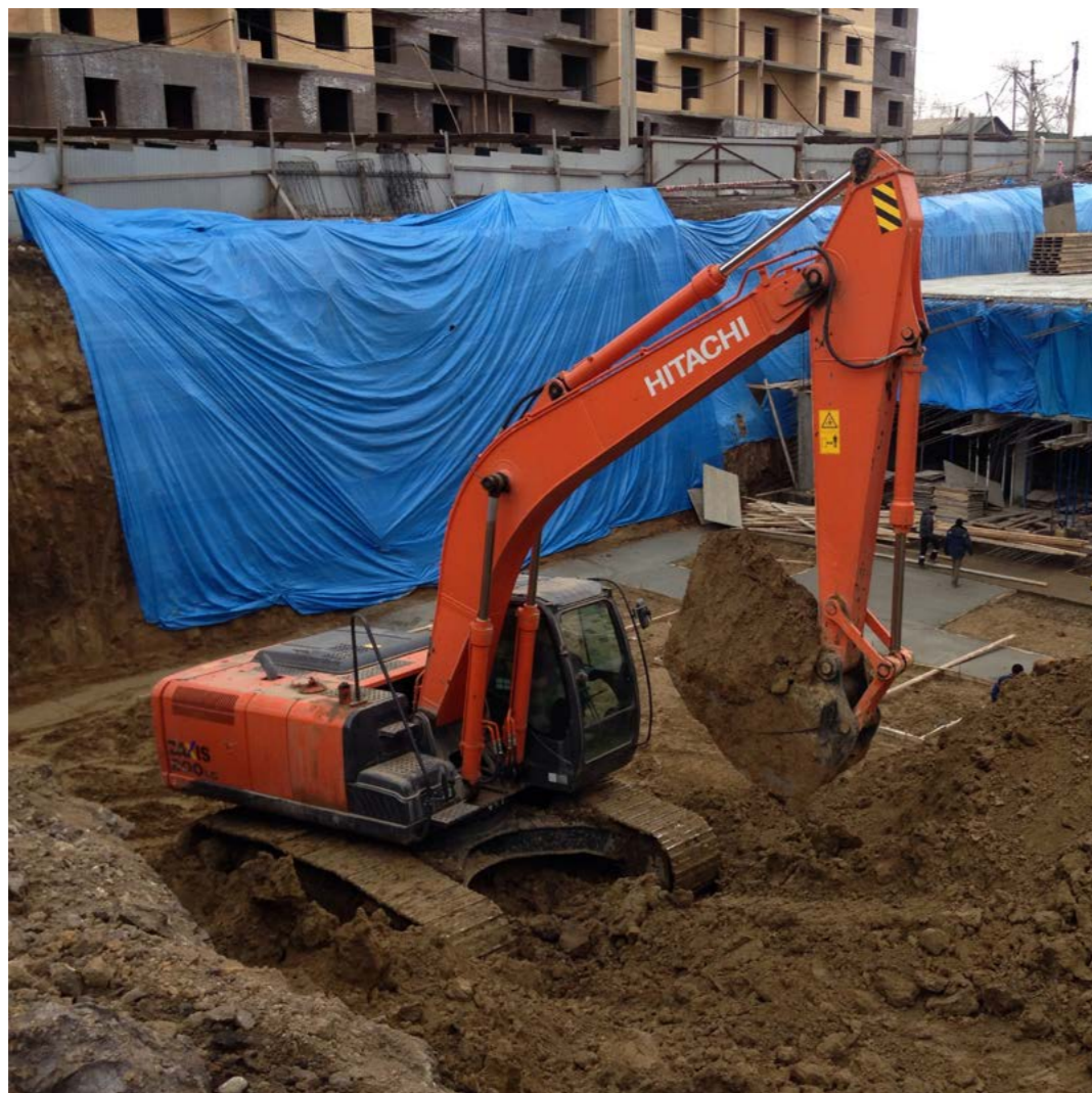
RIPPING BUCKET 0.65 CUBIC METERS/HITACHI ZH200
