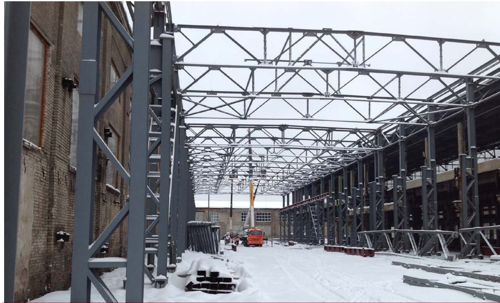
MANUFACTURING AND MOUNTING OF METAL STRUCTURES FOR A PRODUCTION FACILITY OF "PROFESSIONAL" COMPANY, IVANOVO.
