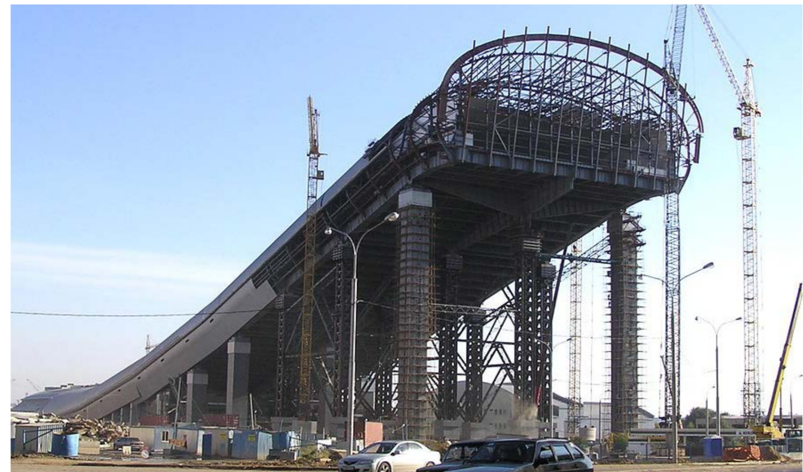
SUPPORT COLUMNS WERE MANUFACTURED FOR A MOUNTAIN SKIING COMPLEX "SNEZH.KOM", KRASNOGORSK, MOSCOW REGION.
